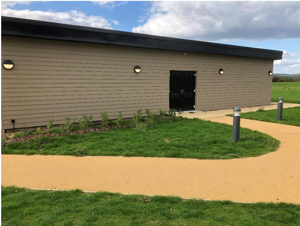
Figure 1 - Changing Facility at Kingley Gate
